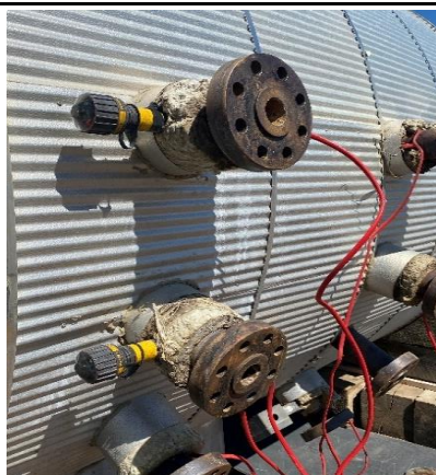
Photo 9: 2" flanges with heat trace in place
