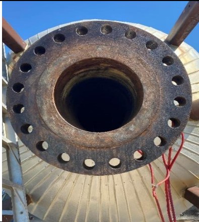
Photo 5: 16" top flange in good condition
