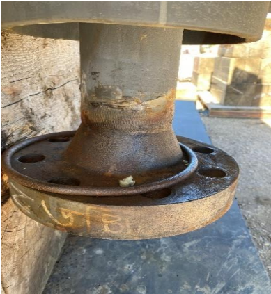
Photo 15: Drain where face damage is present as it exits the skirt
